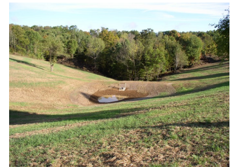
GRADE STABILIZATION STRUCTURE
